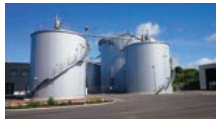
GLS TANKS GLS TANKS INTERNATIONAL GMBH TANK
